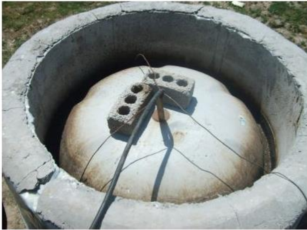
Bioreactor for biogas production at the Golden Wing poultry farm in Bostanlik district of Tashkent region established by Smart Biogaz LLC.
