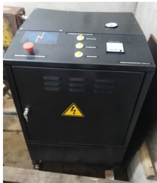
Image 17 After: 35kw New efficient steam generator
