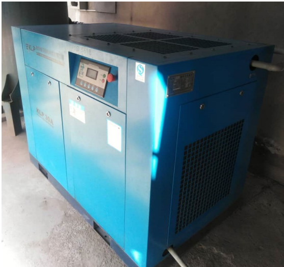
Image 6, After: Cleaned air compressor
