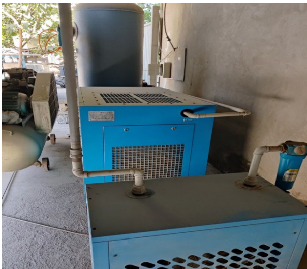
Image 5, Before: Air compressor with accumulated dust
