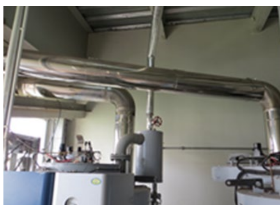
Image 15, After: insulated steam pipeline
