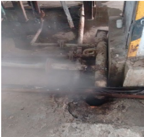
Image 18, Before: Condensate going down the drain
