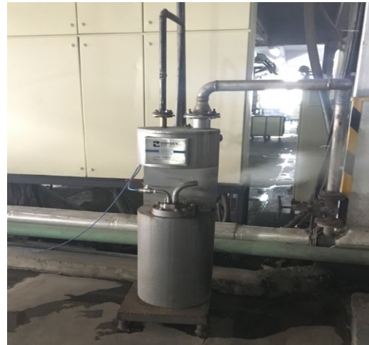
Image 19, After: Condensate recovery system
