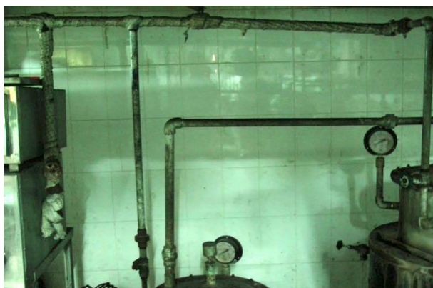
Image 14, Before: Uninsulated steam pipeline
