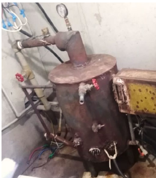
Image 16, Before: 50kW Old steam generator without insulation
