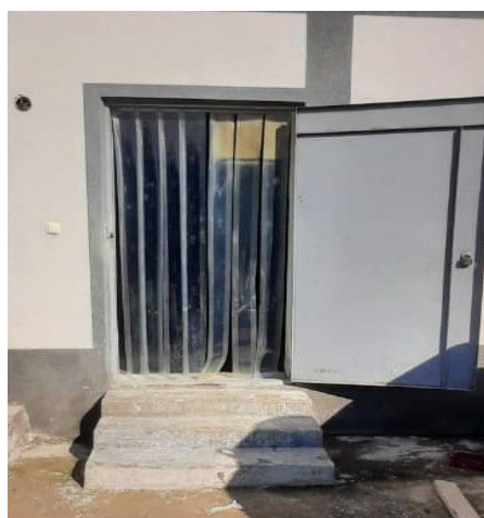
Image 13, After: Cold storage door with PVC curtain
