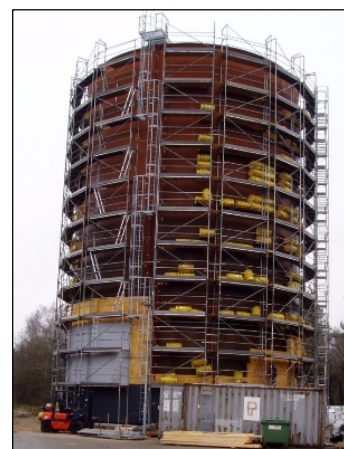
Photo 2.1 Heat accumulator tank under construction. Credit: COWI
