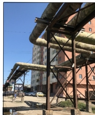
Photo 3.1 Aging piping suggested for replacement. Credit: COWI
