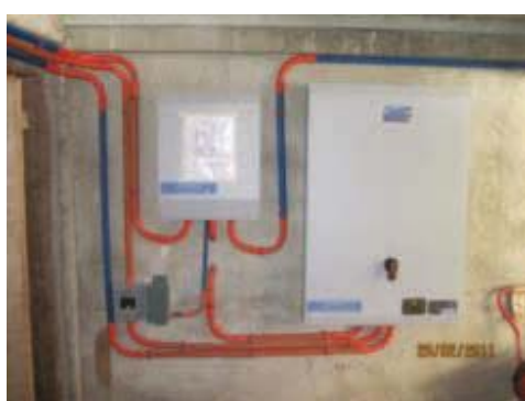
Left Inverter System; Right Solar Charger
