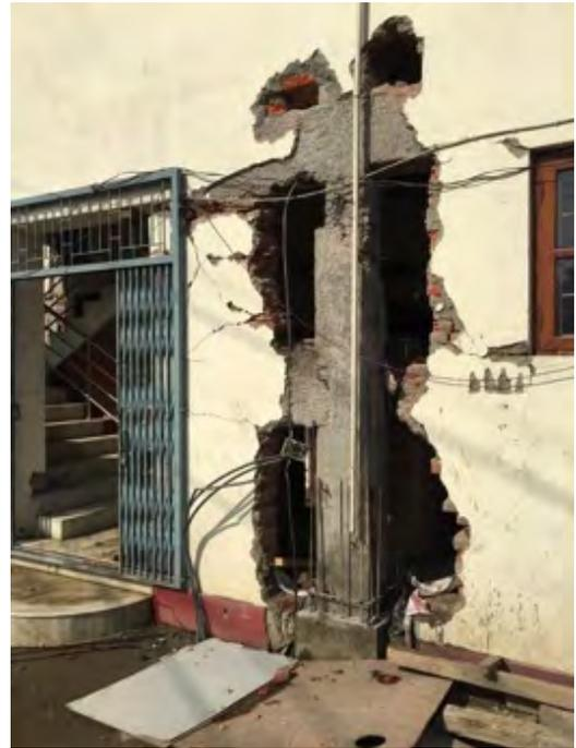
**Image 6: Earthquake damage to Central Carpet Industries Association**
