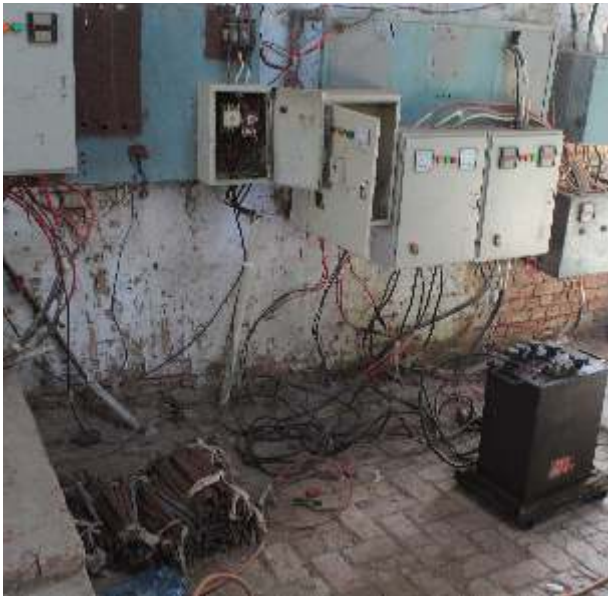
Open electric wiring in ginning hall
