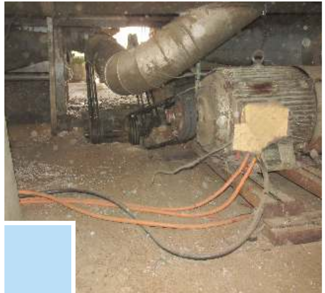
Open electric wiring in ginning hall
