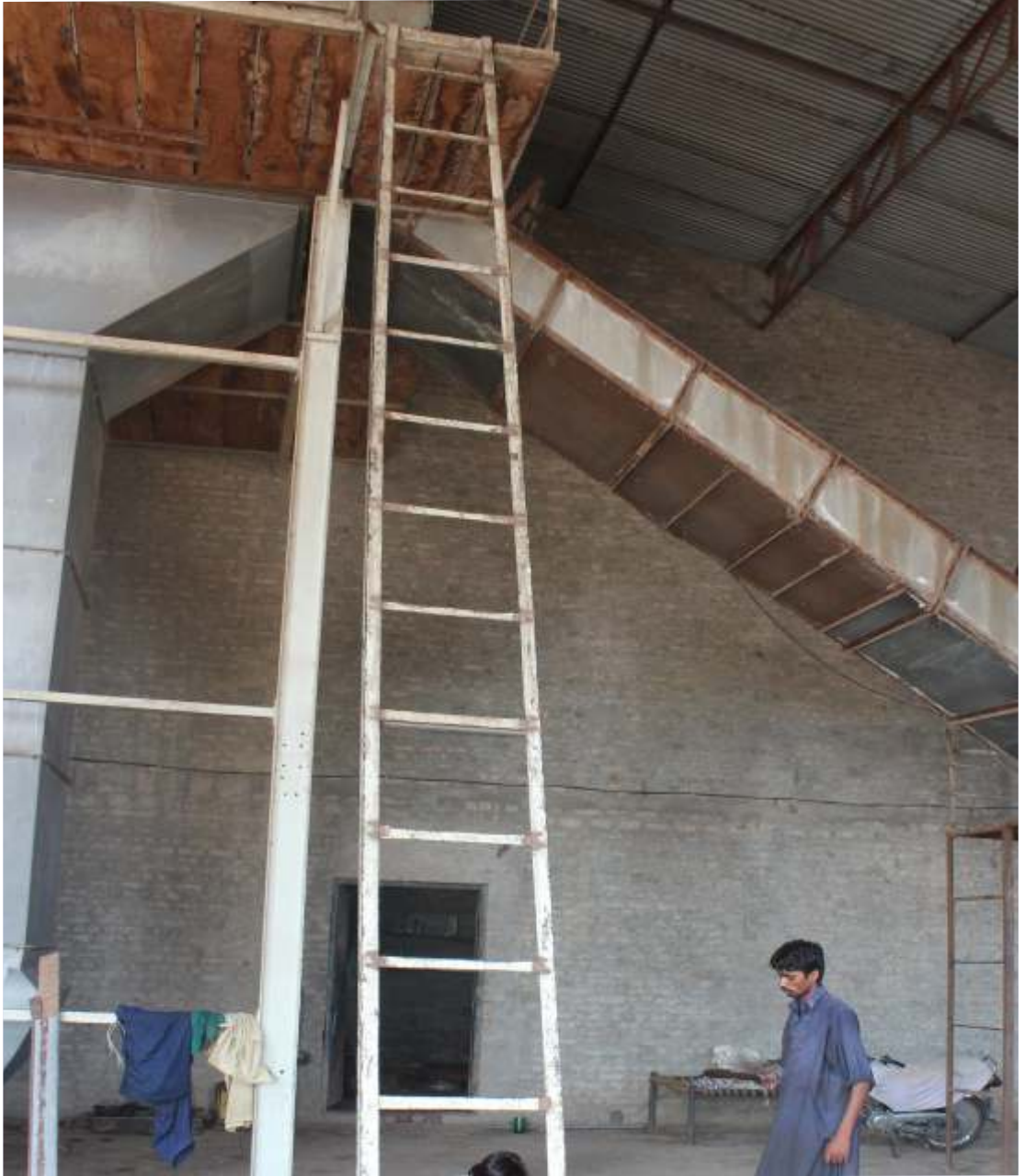
Dangerous ladder used for working up on the platform
