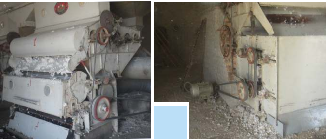
Open Belts Without Protective machine guards
