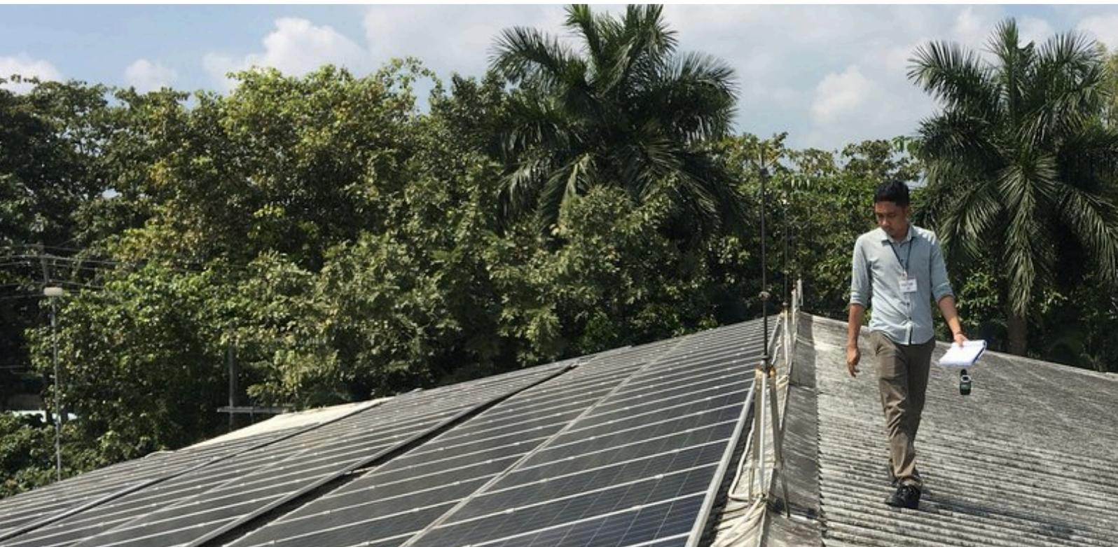
An engineer from SMART Myanmar inspects the solar panels on the first factory in Myanmar to implement rooftop solar, a garment manufacturer in Yangon. Since this factory's 80 kW system was installed another five garment factories have also implemented solar PV. The largest of these systems has a rated peak generation capacity of 250 kW.
