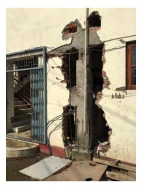
Image 6: Earthquake damage to Central Carpet Industries Association
