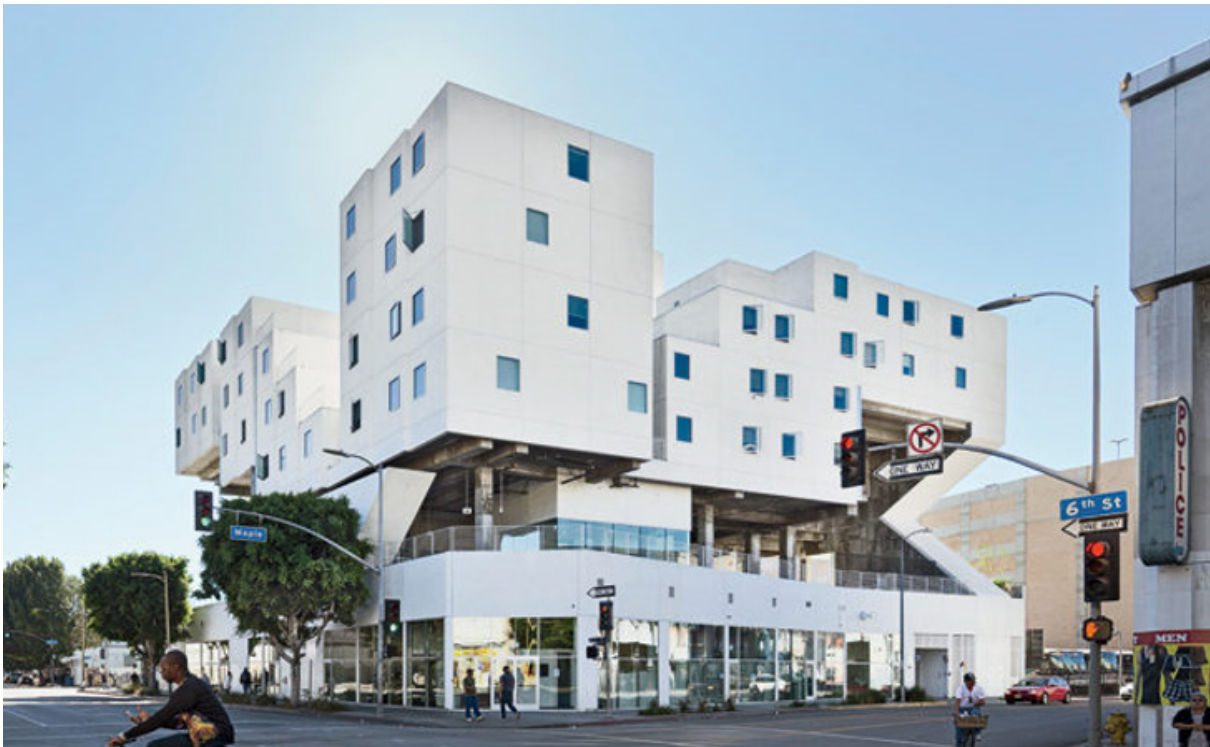
Figure 6: Star Apartments in Los Angeles
