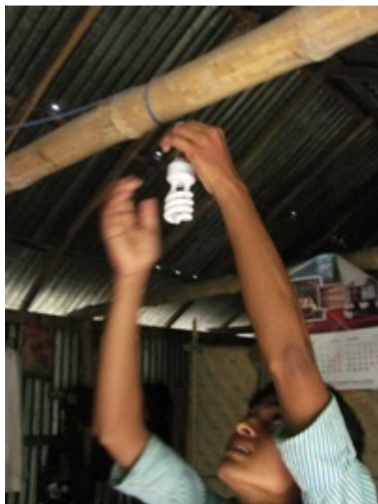
Figure 5: Installation of CFL bulbs
