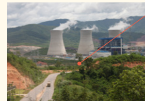
Hongsa lignite power plant (1,878 MW)
