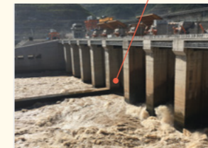
Xayaburi dam (1,285 MW)
