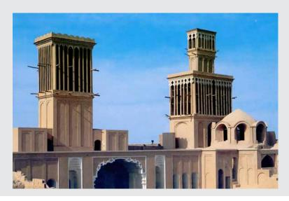
FIGURE 23. Central wind tower with water for cooling for use in hot and dry climates (Image from Kamal, 2012)<sup>127</sup>
