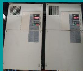
Output speed of 44 nos. of motors is now controlled through variable frequency drives (VFD). This improves productivity (as VFD setting change is faster and easier than changing pulleys) and significantly reduces the energy used at lower speeds of operation.
