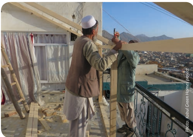
Building the Veranda
