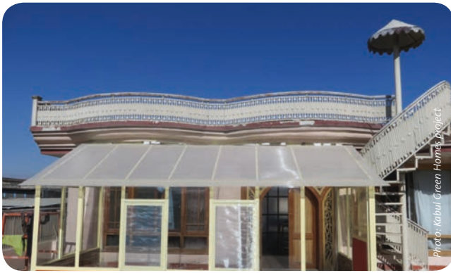
Veranda covered by glas
