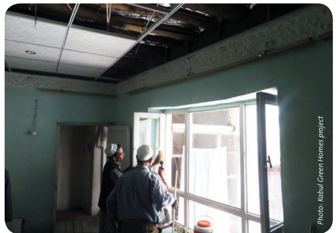
Double glazing and ceiling insulation installation
