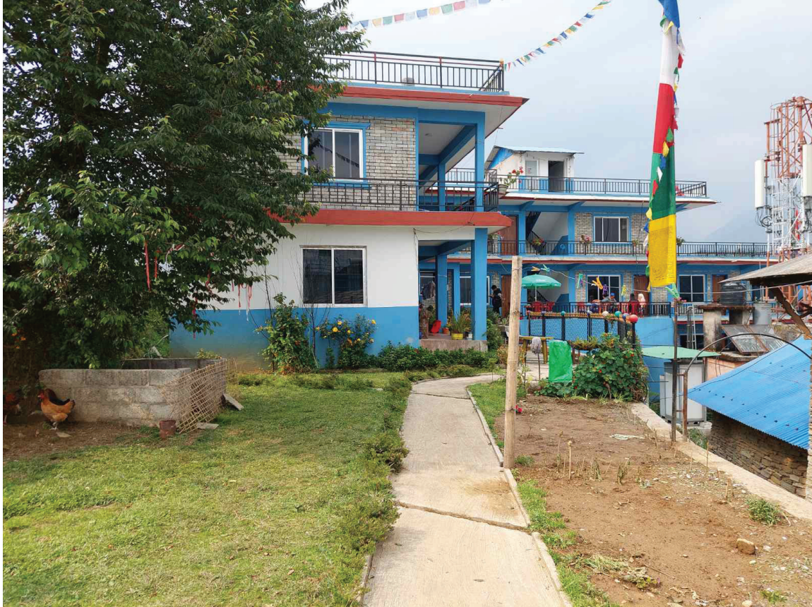
Figure 85: Hotel Building at Annapurna Rural Municipality
