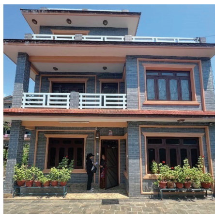
Figure 11: House surveyed at Pokhara SMC (Source: Urban Park)
