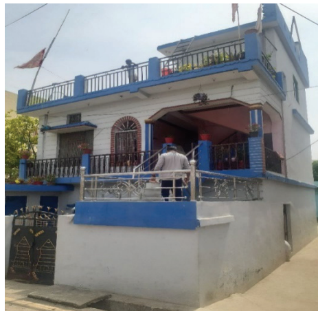
Figure 9: Surveyed house at Nepalgunj (Source: Urban Park)
