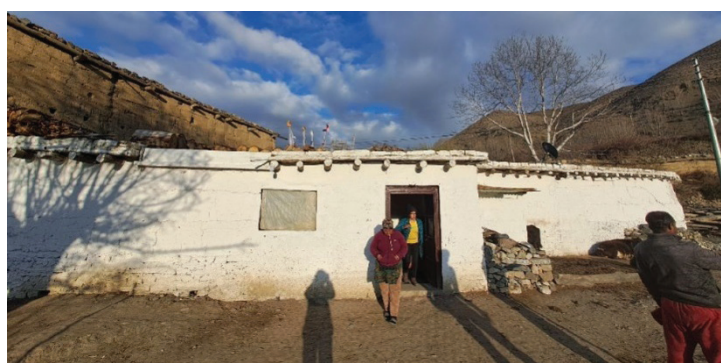
Figure 14: Surveyed house at Varahung Muktichhetra (Source: Urban Park)
