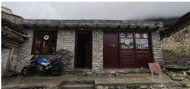
Figure 13: Surveyed House at Gharapjhong (Source: Urban Park)
