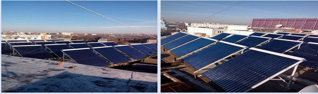
Figure 15. Residential 9-storey building, Tashkent, Mirobad district, Oybek street 42.
